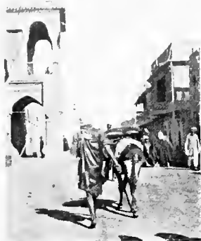
ENTRANCE TO ASHAR BARRACKS.
